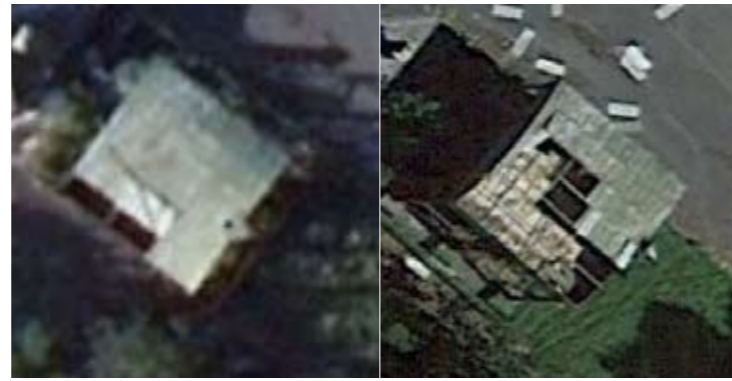
Picture 17 & 18: Building 4. Aerial photos show that a significant amount of the vaulted roof covering has been removed since 2016. More than half has been stripped.
