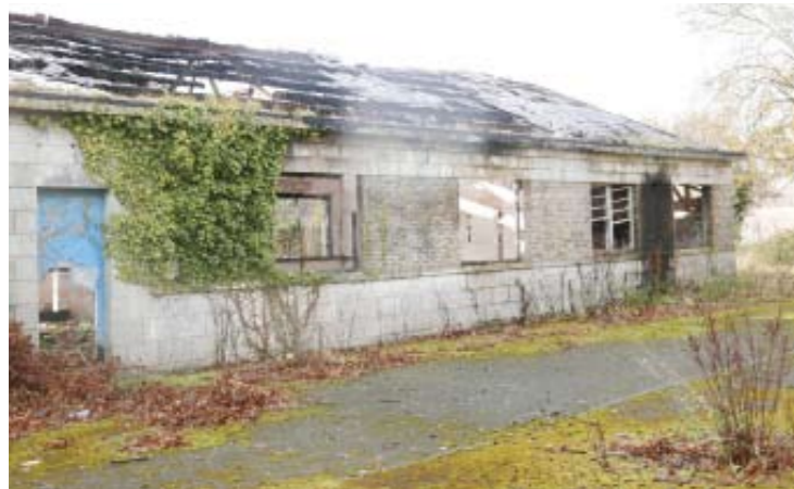
Picture 8: Building 1, NCO's mess. The west end of which is burnt out
