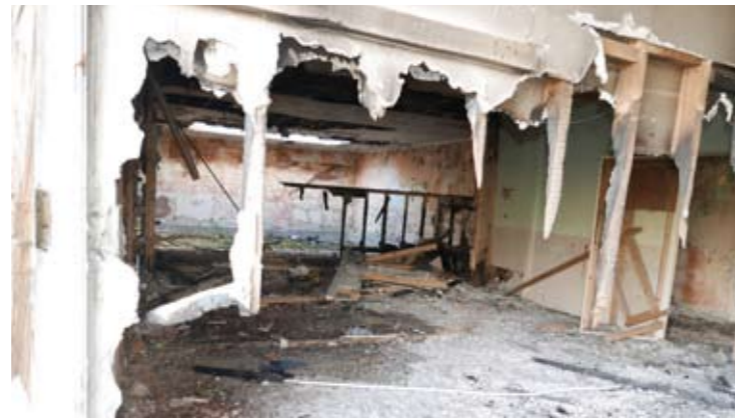
Picture 13: Building 1, Interior of the NCO's mess
