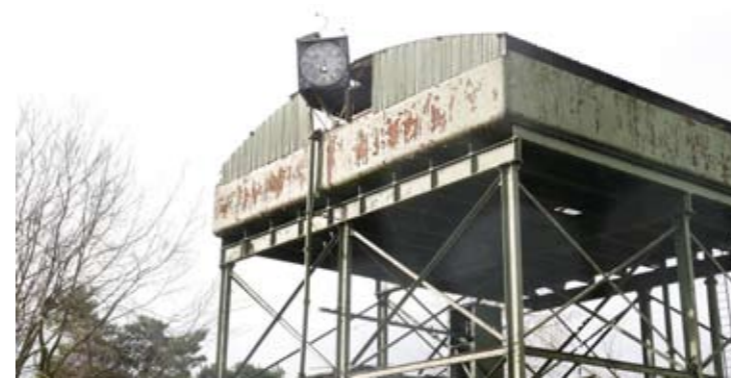
Picture 19: Building 4. The tank and clockface.
