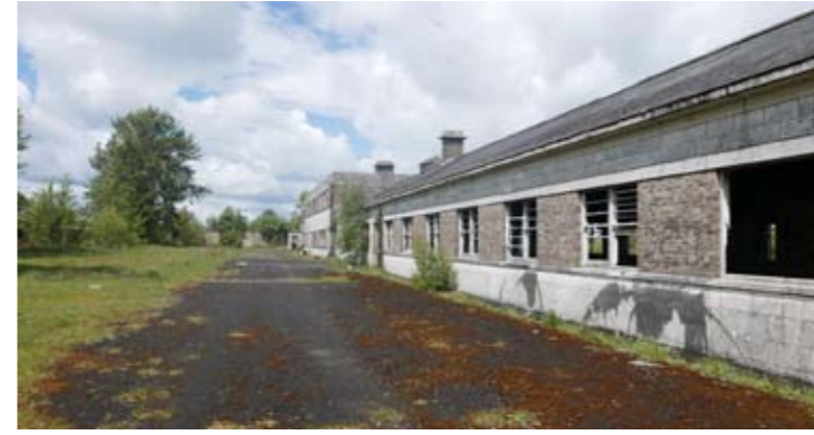
Picture 2: Building 1. The former NCO's Mess, constructed of concrete block and brick walls with a pitched gabled and slated roof.
