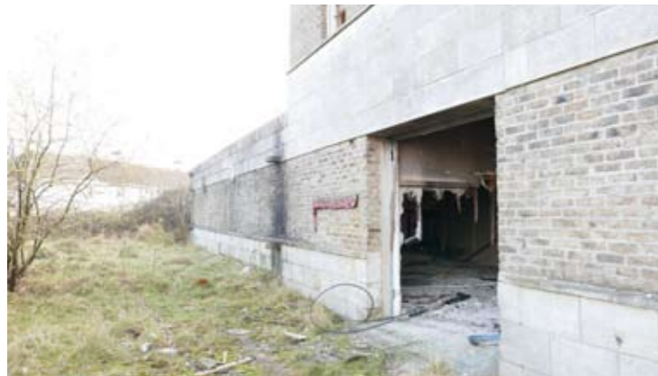
Picture 12: Building 1. NCO's mess
