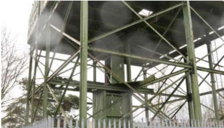
Picture 21: Building 4, support structure
