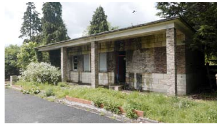
Picture 26: Building 5 which is a security building or gate house at the entrance gates
