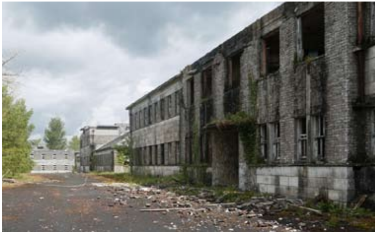
Picture 67: Building 13 with building 14 and building 18 beyond
