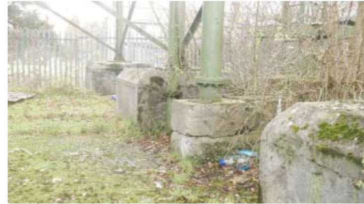
Picture 23: Building 4, foundations
