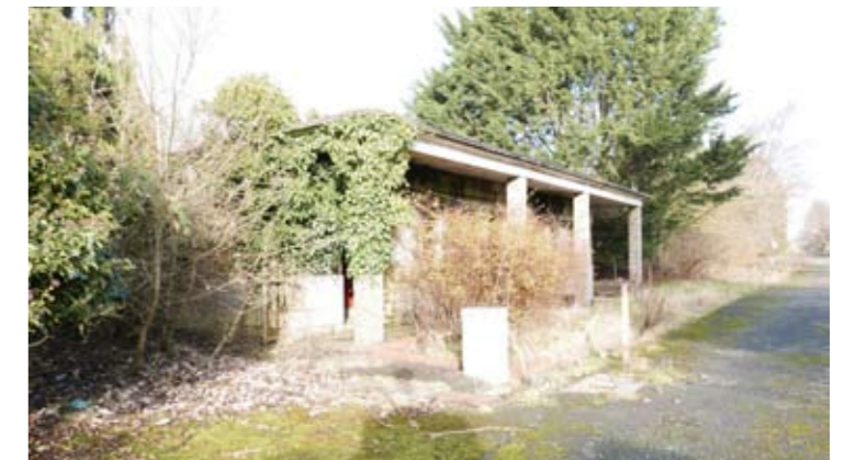
Picture 27: Building 5 which is a security building or gate house
