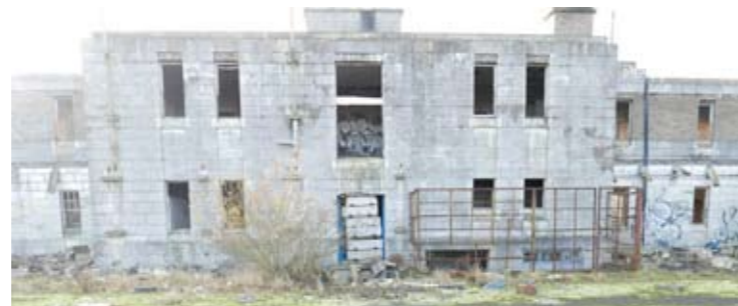
Picture 41: Building 9. Detailed view of the rear or north elevation of the Officer's Mess building shows that it has been subject to vandalism and neglect and has suffered a loss of character
