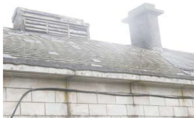
Picture 9: Lantern to Building 1
