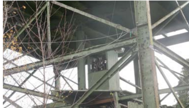
Picture 22: Building 4, support structure
