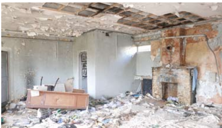
Picture 28: Building 5 interior
