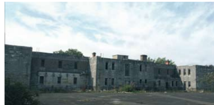
Picture 38: Building 9. Rear or north elevation of the Officer's Mess building
