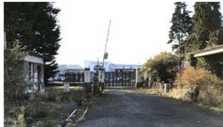
Picture 25: Building 6 (l) and building 5 (r) Looking back towards entrance gates
